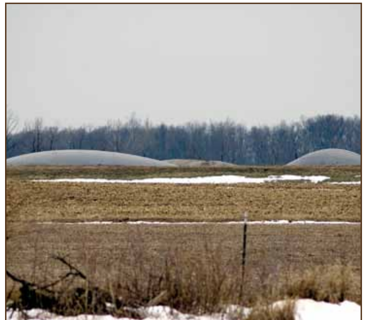
Gas bubbles in the liner of the Union Go Dairy manure lagoon in Randolph County, Indiana. Photo by BloomingtonAlternative.com.
